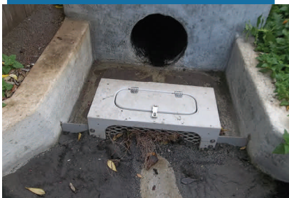
Flume filter box, 14th Street, Montara
