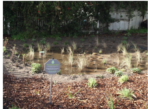
Rain garden installed for biofiltration of runoff in the ASBS watershed
