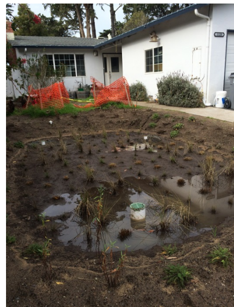
Rain garden during construction, Montara
