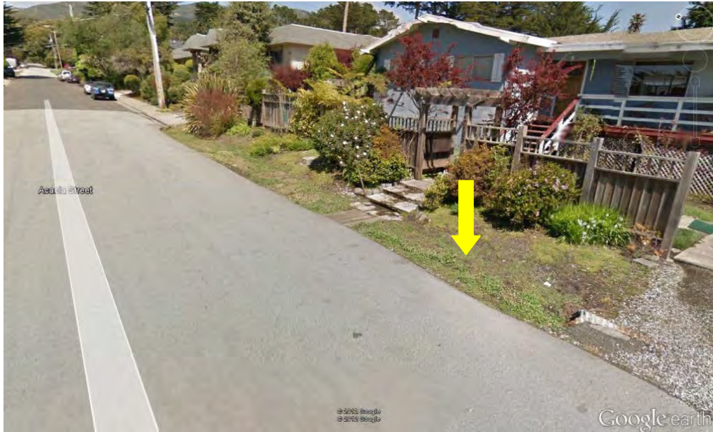
Photo 18: DITCH-9 ~ Acacia St at Kanoff St (P-MN-F-L030-120)
