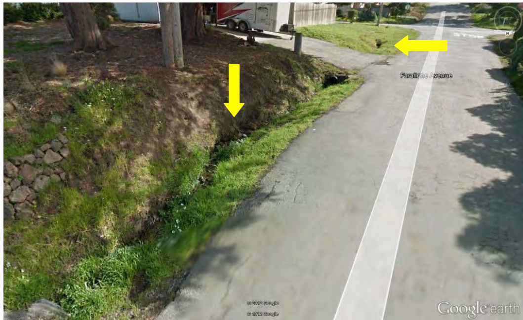
Photo 11: DITCH-2 ~ Farallon Ave and 4 th St (P-MN-C-120)
