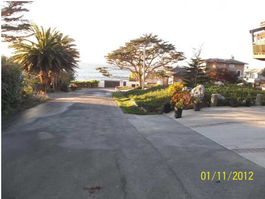
FIT003-A_01112012: 7 th St Post-construction
