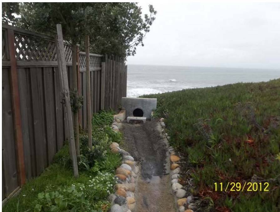
FIT009-B_11292012: 14 th St North Post-construction
