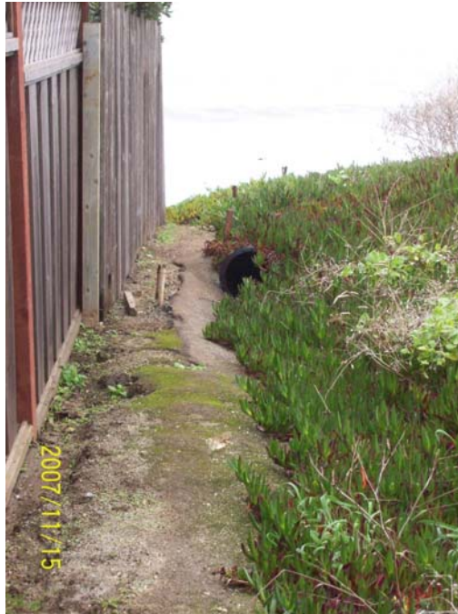
FIT009-A_11152007: 14 th St North Pre-construction
