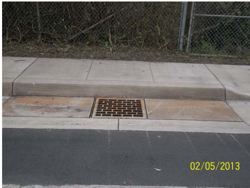
NLAKE -B_02052013: North Lake St Post-construction
