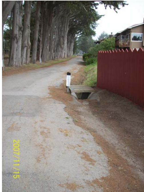
FIT027-A_11152007: Cypress Ave Pre-construction
