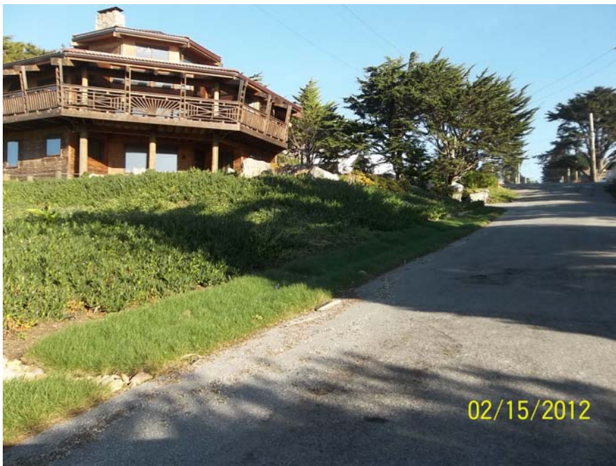
FIT003-B_02152012: 7 th St Post-construction
