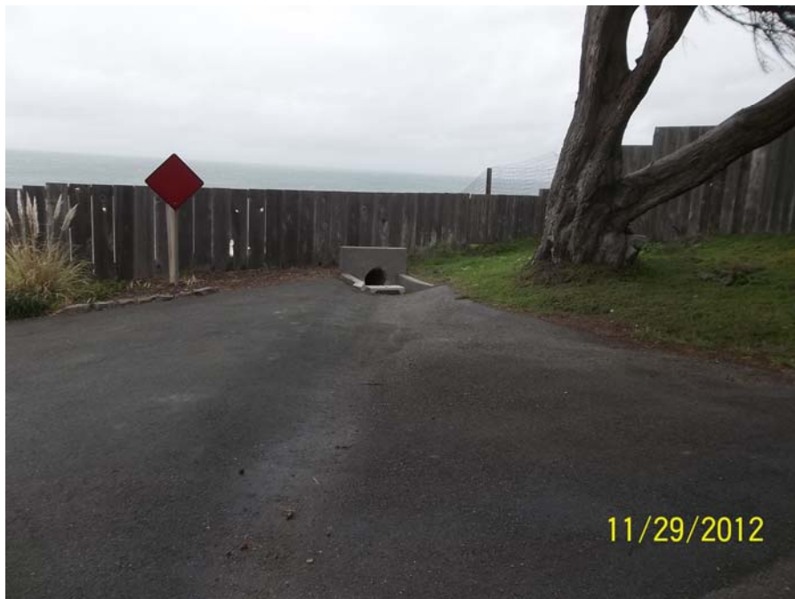
FIT002-B_11292012: Seacliff Ct Post-construction
