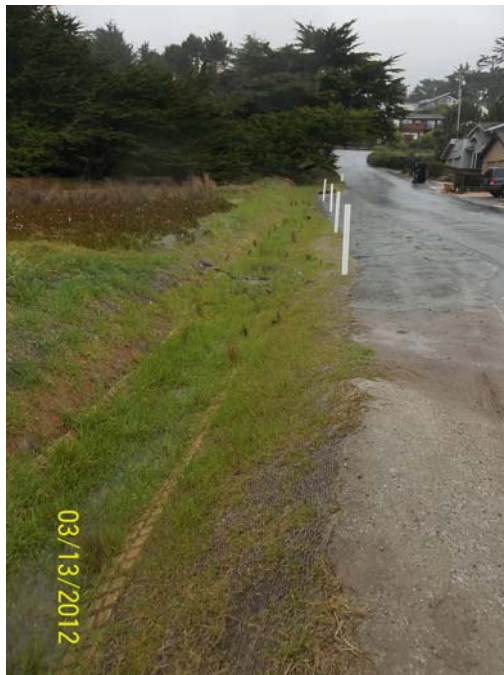
FIT015-A_03132012: Juliana Ave Post-construction
