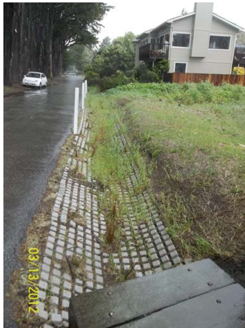
FIT027-A_03132012: Cypress Ave Post-construction
