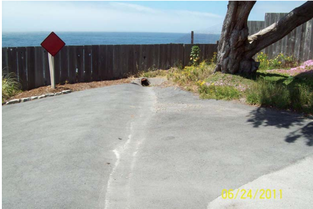
FIT002-B_06242011: Seacliff Ct Pre-construction
