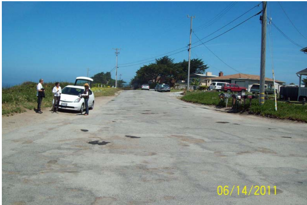
FIT029-A_06142011: Ocean Blvd Pre-construction
