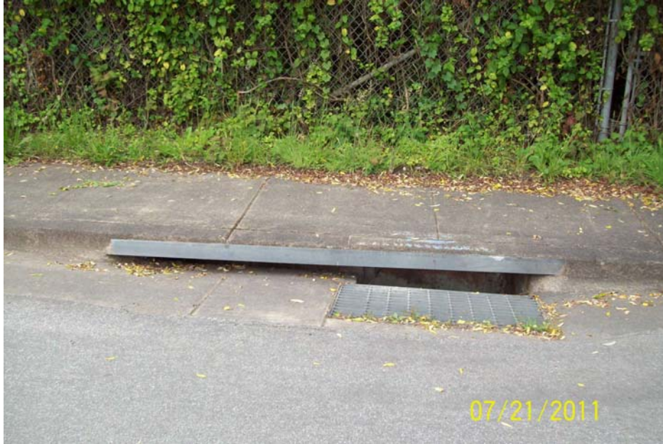
NLAKE -B_07212011: North Lake St Pre-construction
