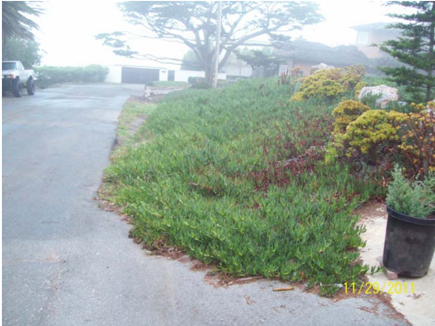
FIT003-A_11292011: 7 th St Pre-construction
