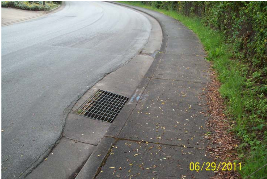
NLAKE-A_06292011: North Lake St Pre-construction
