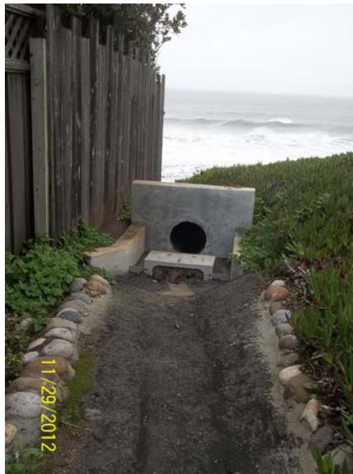
FIT009-A_11292012: 14 th St North Post-construction
