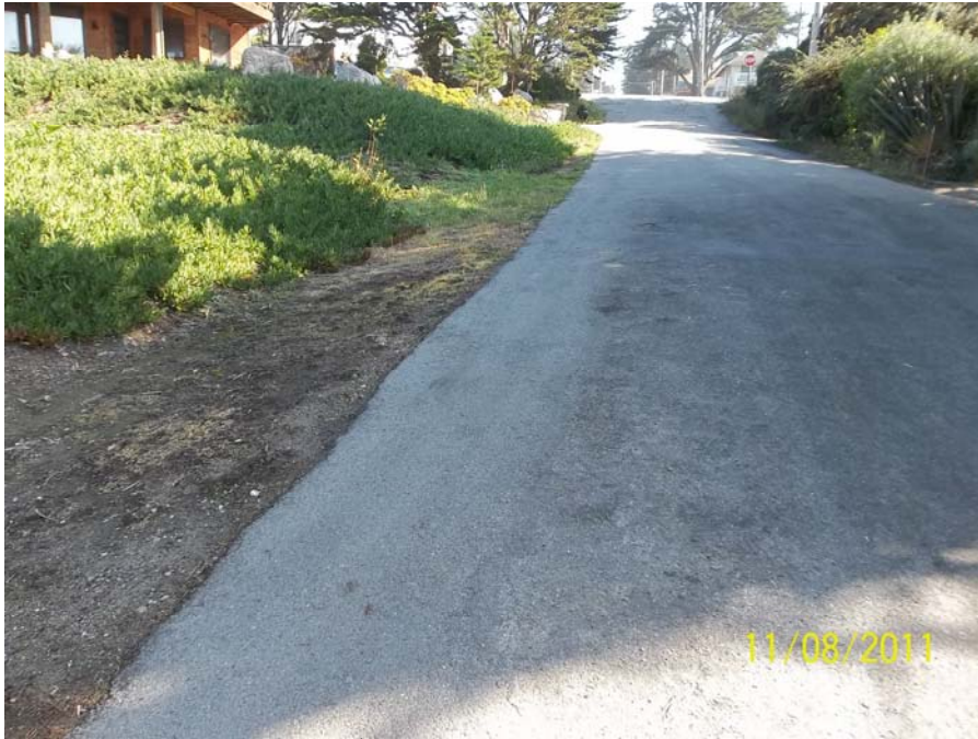
FIT003-B_11082011: 7 th St Pre-construction
