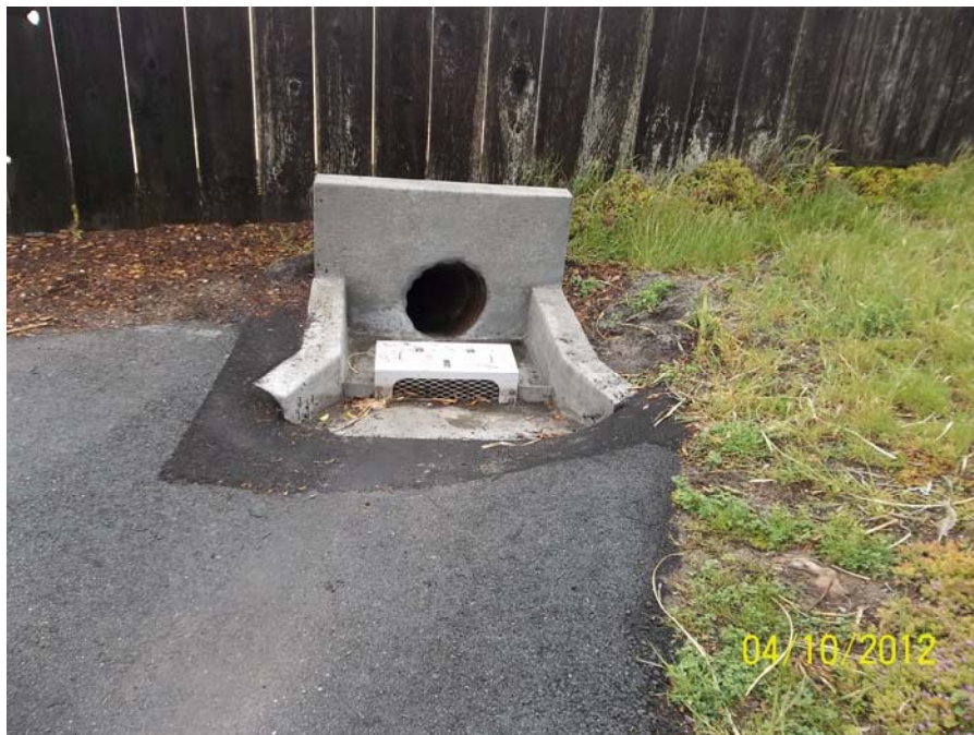
FIT002-A_04102012: Seacliff Ct Post-construction
