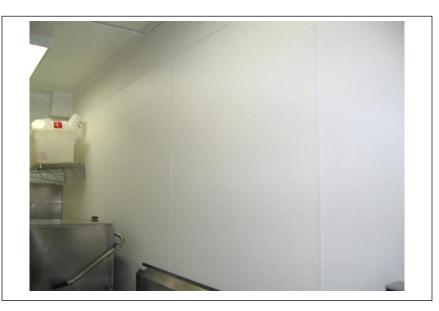
Typical FRP installation behind wall surface of sinks and prone splashing areas.
