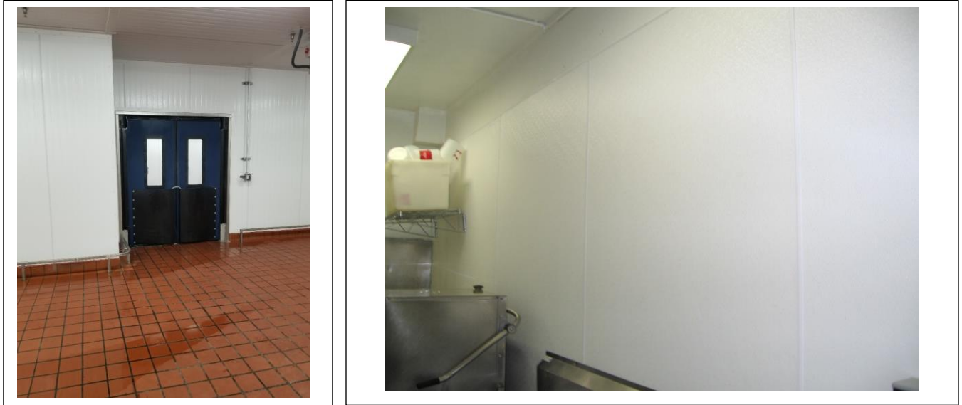
Typical FRP installation behind wall surface of sinks and prone splashing areas.
