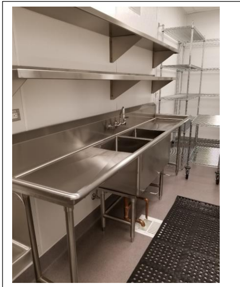
Indirect waste drain connection (floor-sink flushed to the floor)
