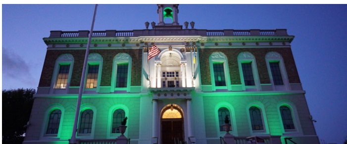
City Hall, South San Francisco
