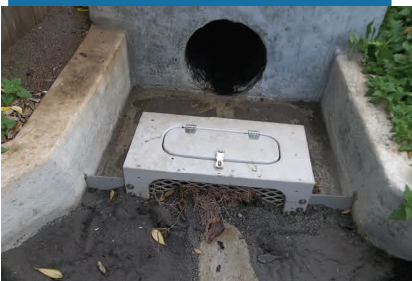
Flume filter box, 14th Street, Montara
