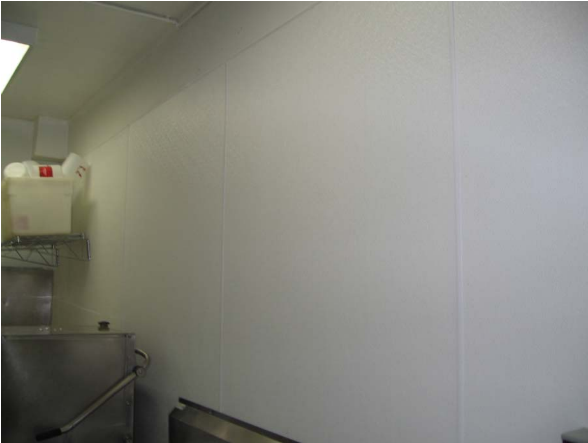
Typical FRP installation behind wall surface of sinks and prone splashing areas
