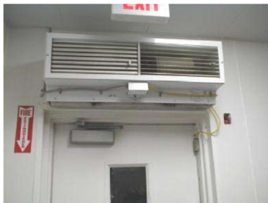
Typical air curtain installation.
