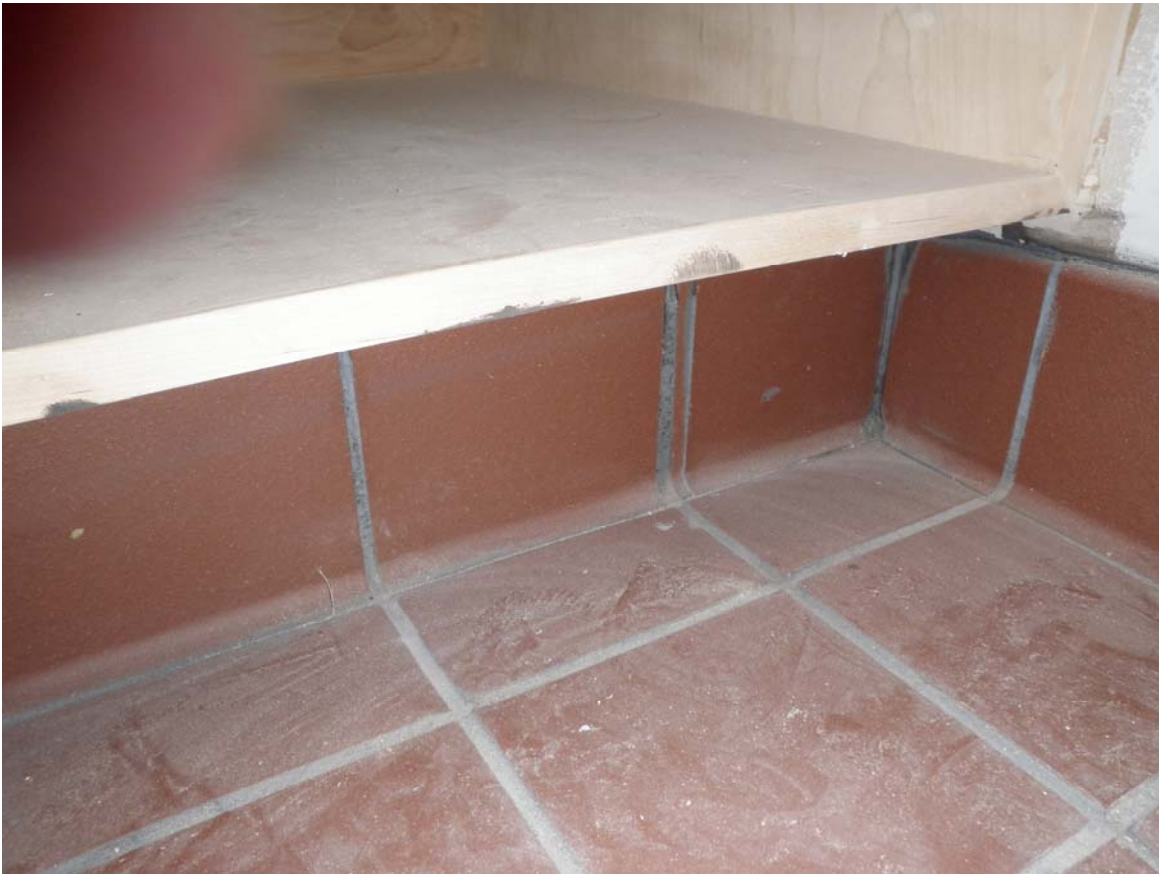
Typical Quarry tile with 3/8" radius coving
