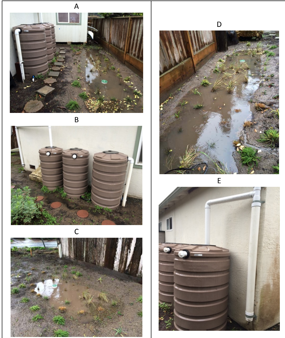
Figure 6. Examples of rain barrels installed in the vicinity of the James V Fitzgerald Marine Reserve. A) Private rain barrel and rain garden system in Moss Beach, CA; B) and C) Front yard rain barrels with rain garden; D) and E) Back yard rain garden and rain barrels connected to down spout.
