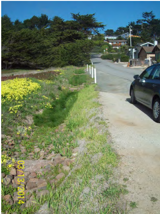
Figure 12. Juliana Avenue vegetated swale.
