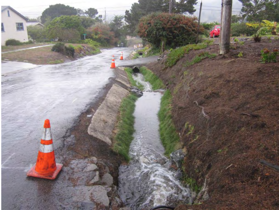
Figure 6. Farallone Avenue @ 4th Street vegetated swale.
