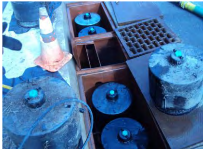
Clean catch basin with new filters added
