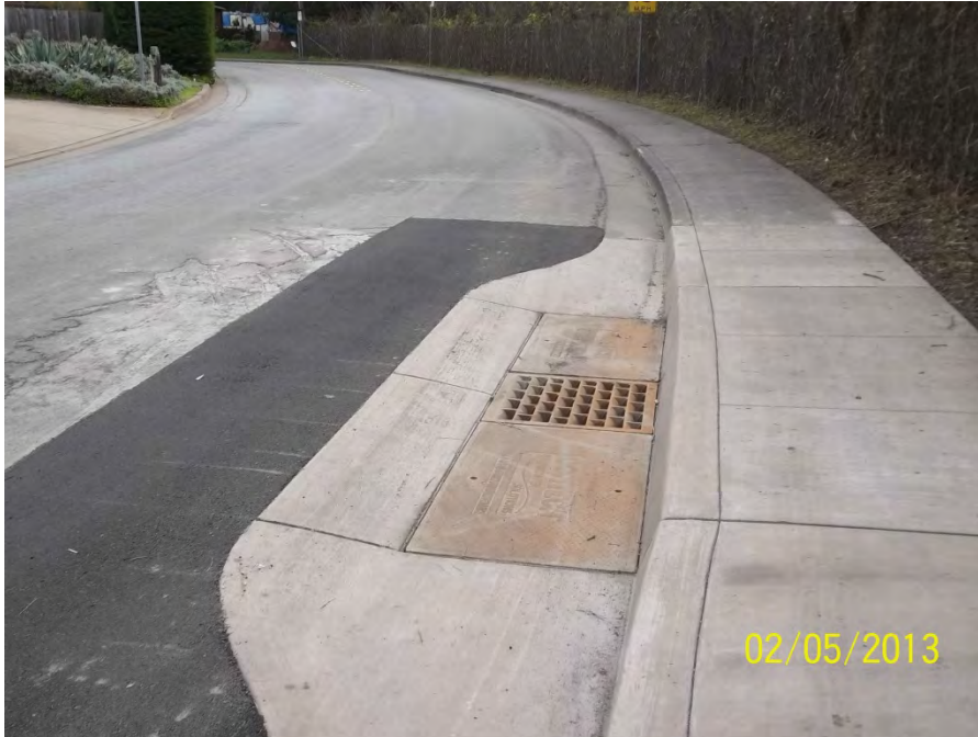
Figure 19. North Lake Street StormFilter system.
