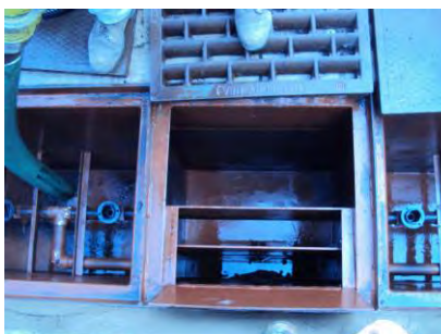
All sediment removed from inlet bay of Catch Basin
