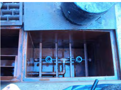
All sediment removed from inlet bay of Catch Basin
