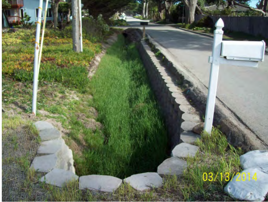
Figure 14. Wienke Way vegetated swale.
