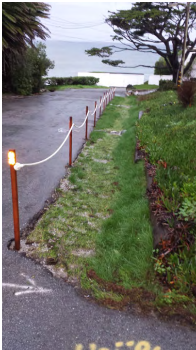
Figure 3. 7th Street vegetated swale along north side of roadway.
