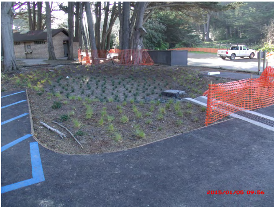
Figure 18. Fitzgerald Marine Reserve Parking Lot bioretention system.
