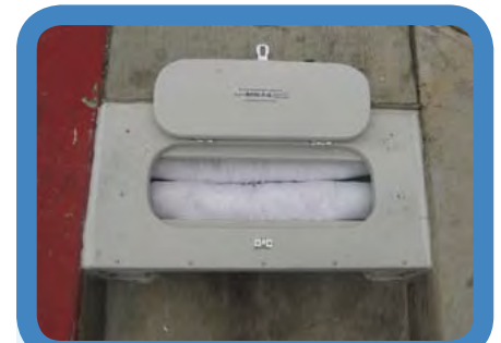
Access Hatch for Easy Media Replacement
