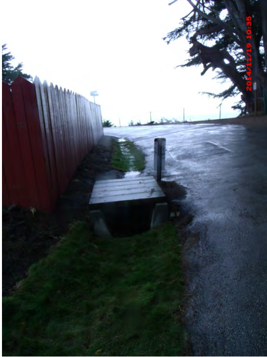
Figure 21. Cypress Avenue vegetated swale (west segment).
