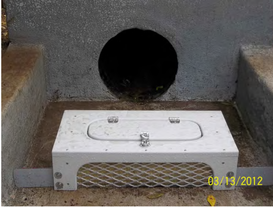
Figure 11. 14th Street south flume filter box.
