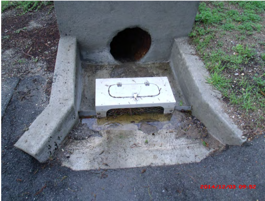
Figure 1. Seacliff Court flume filter box.
