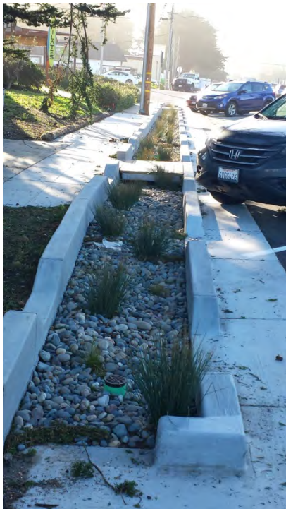
Figure 16. Southern segment of Carlos Street bioretention system.
