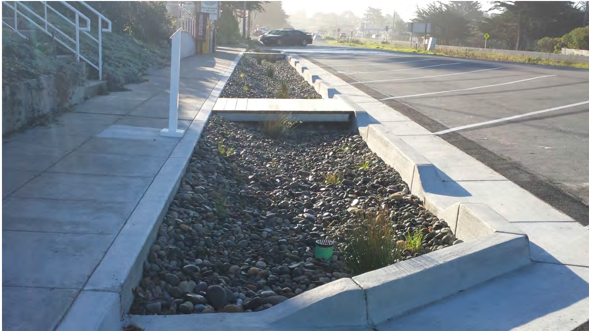
Figure 15. Northern segment of Carlos Street bioretention system.
