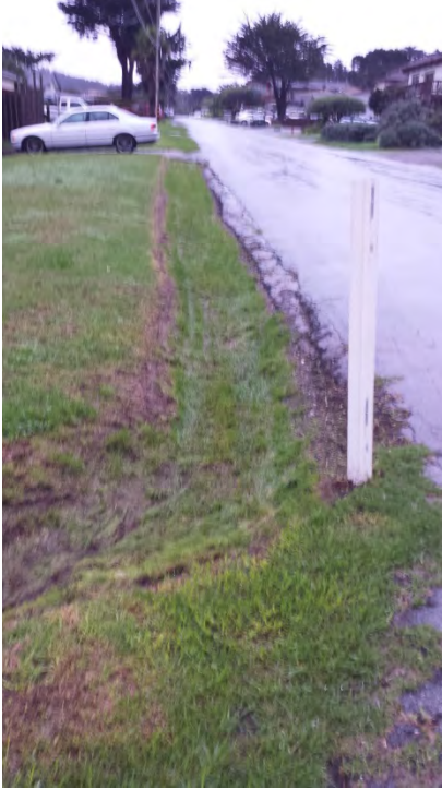
Figure 7. 4th Street vegetated swale.
