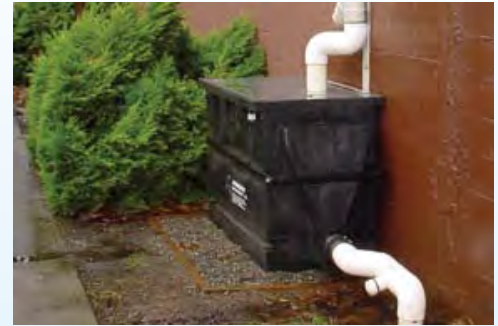
DownSpout StormFilter
