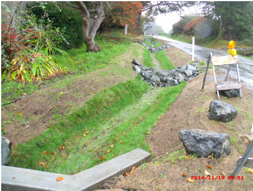
Figure 5. Farallone Avenue @ 3rd Street vegetated swale.
