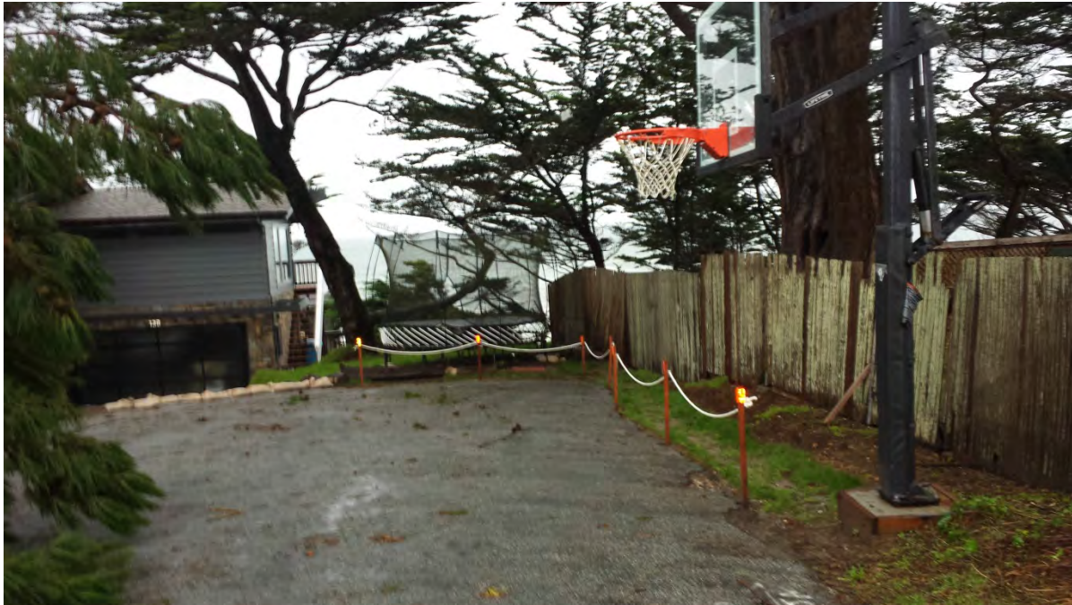
Figure 9. 11th Street vegetated swale.
