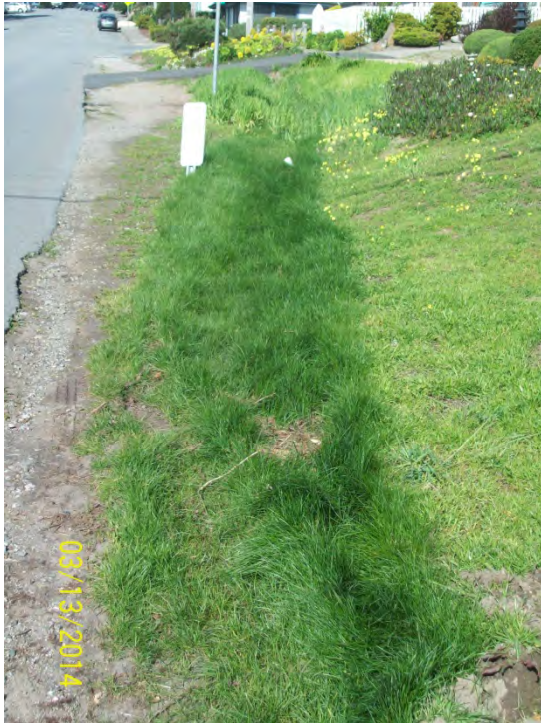
Figure 8. Main Street vegetated swale.
