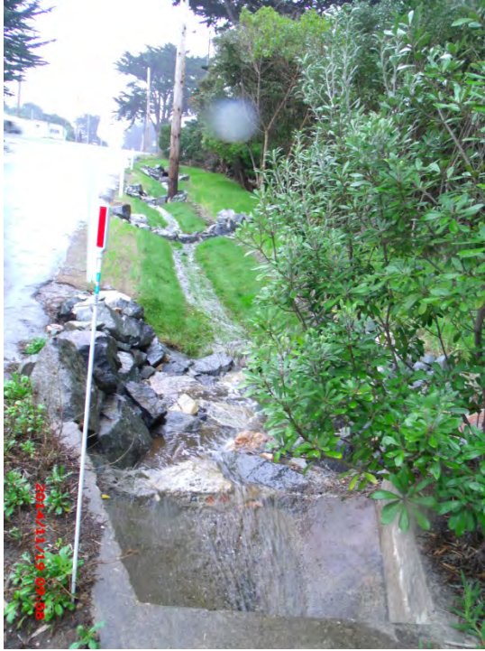
Figure 4. 7th Street swale along south side of roadway.
