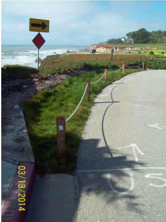
Figure 13. Juliana Avenue vegetated swale.
