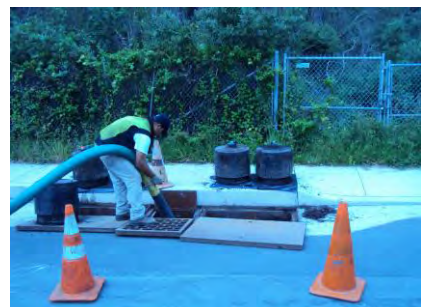
Spent filters removed sediment removal
