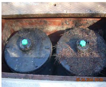
Scumline above top of filter cartridge
