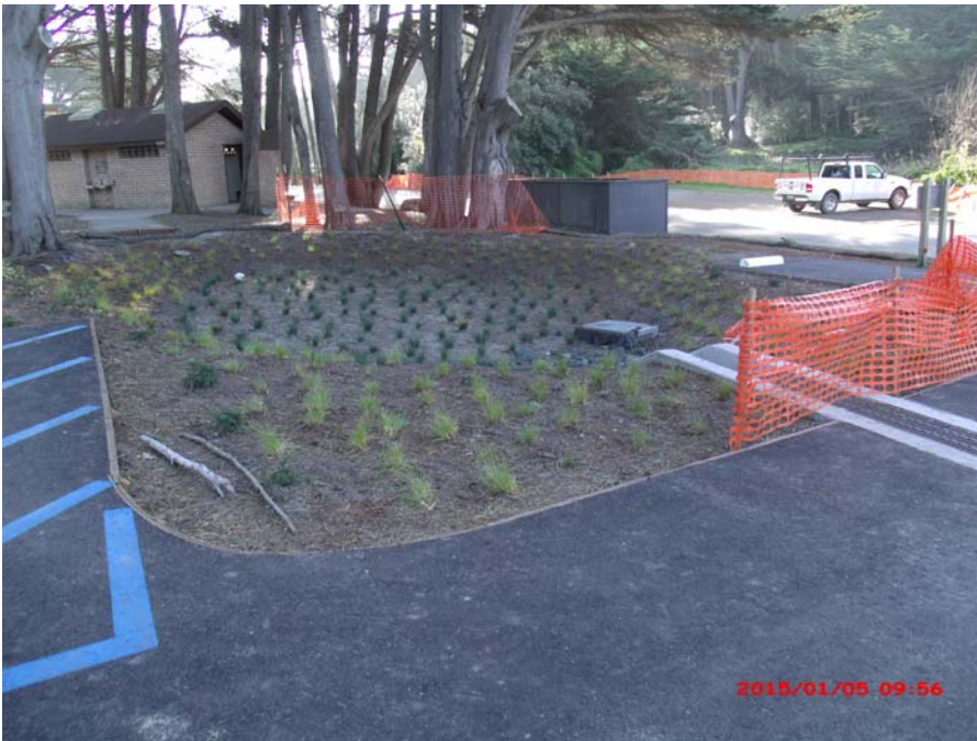
FIT025-B_01052015: Fitzgerald Marine Reserve Parking Lot Post-construction
