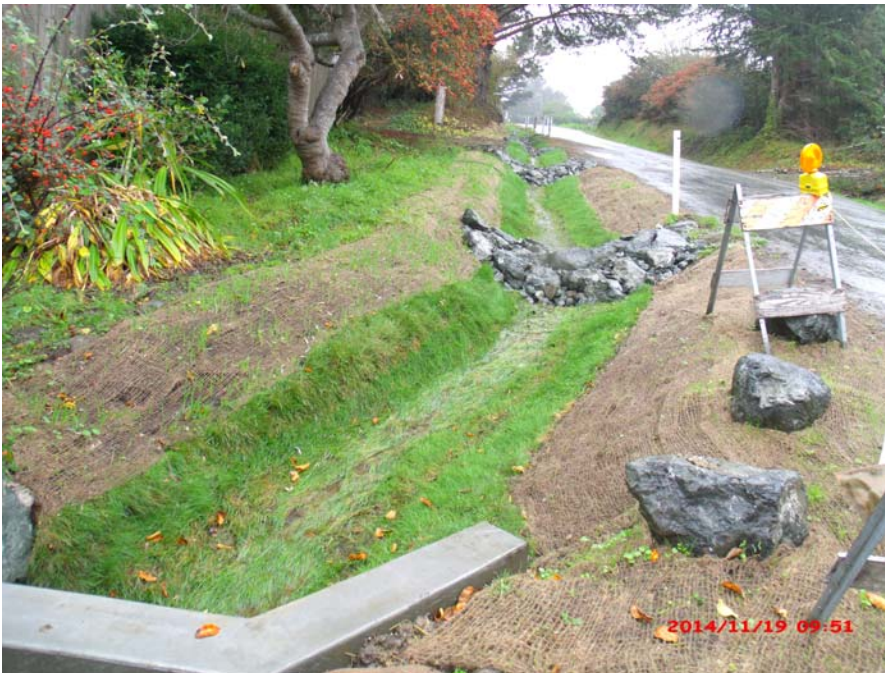
KAN001a-B_11192014: Farallone Ave @ 3 rd St Post-construction
