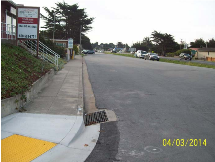
FITNEW1b-A_04032013: Carlos St Pre-construction
