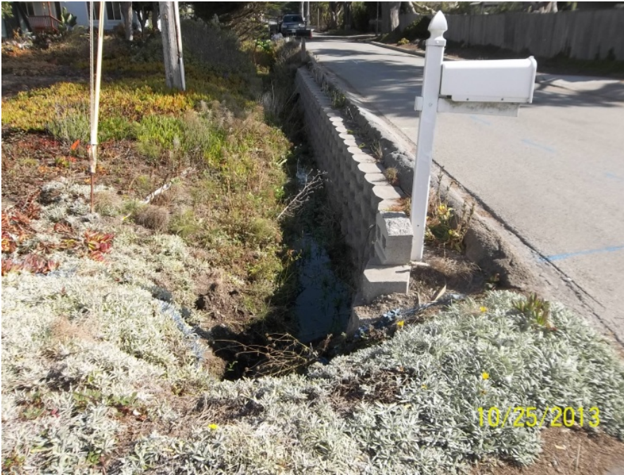
FITNEW1a-A_10252013: Wienke Way Pre-construction
