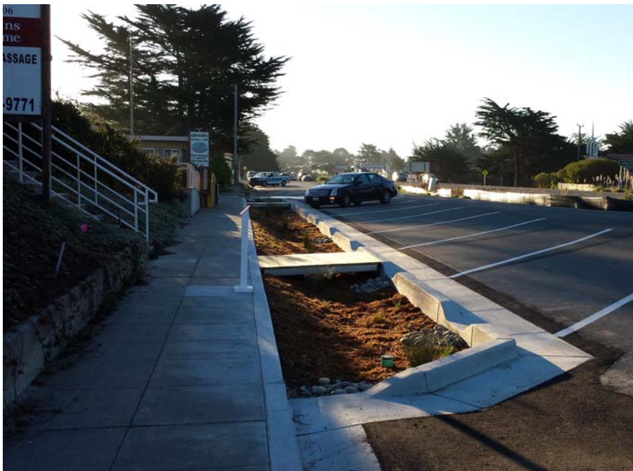
FITNEW1b-B_01062015: Carlos St Post-construction
