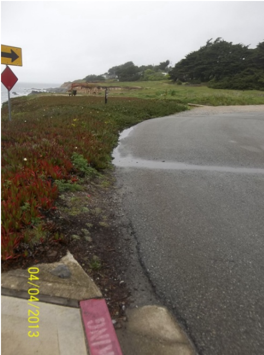
FIT015b-A_04042013: Juliana Ave (lower) Pre-construction
