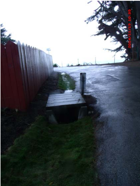
FIT027b-B_111914: Cypress Ave (lower) Post-construction
