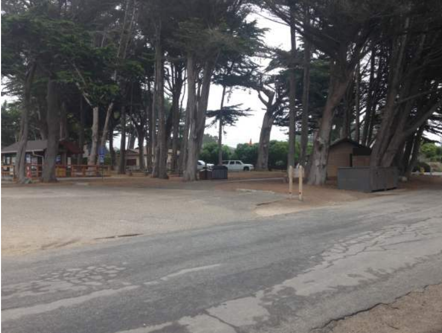
FIT025-A_092014: Fitzgerald Marine Reserve Parking Lot Pre-construction
