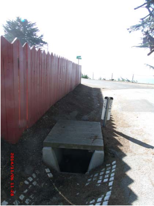
FIT027b-A_11062014: Cypress Ave (lower) Pre-construction
