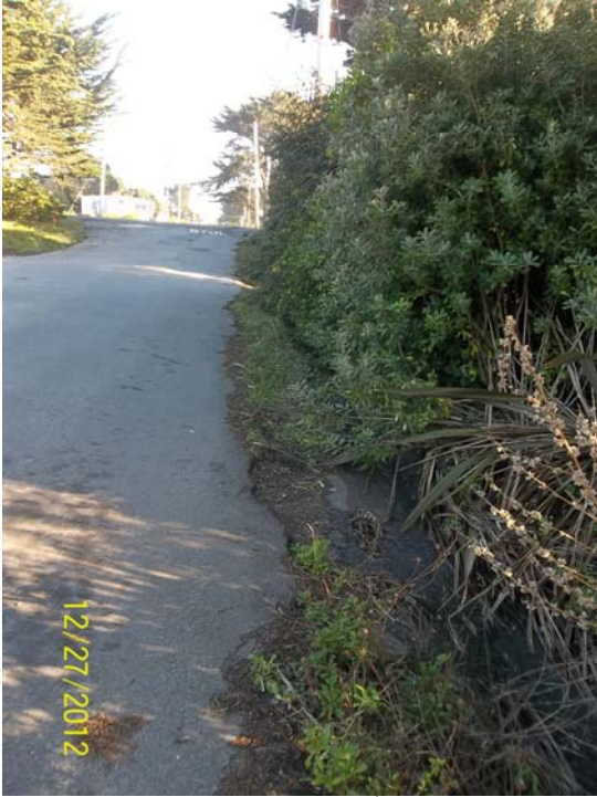
FIT003b-A_12272012: 7 th St Pre-construction
