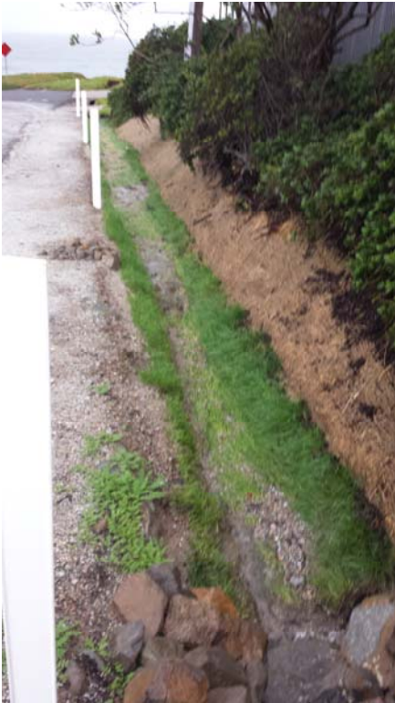
FIT008-B_12122014: 14 th St Post-construction
