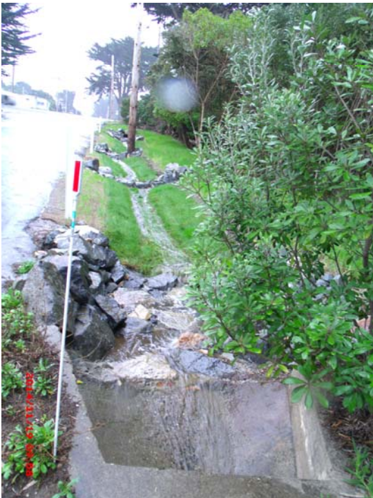
FIT002b-B_11192014: 7 th St Post-construction
