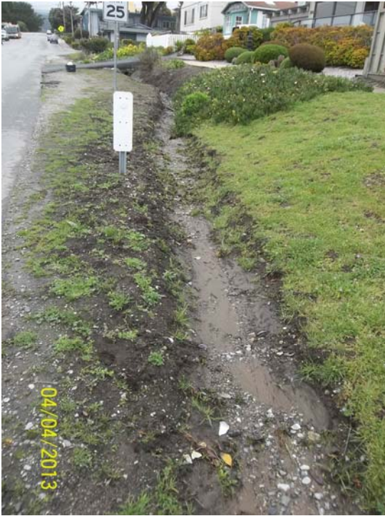
MAIN-A_04042013: Main St Pre-construction
