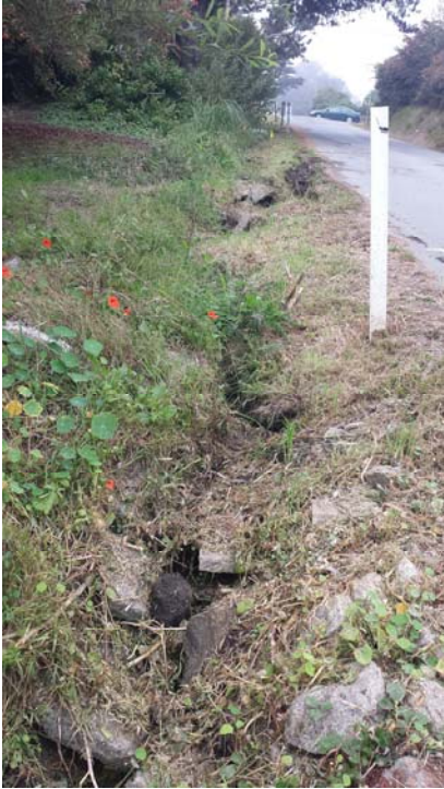
KAN001a-A_10062014: Farallone Ave @ 3 rd St Pre-construction
