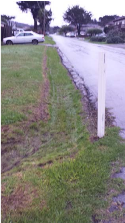
KAN001c-B_12122014: 4 th St Post-construction
