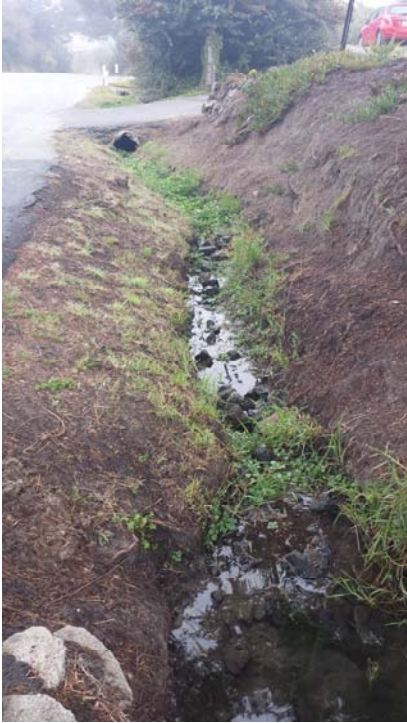
KAN001b-A_10062014: Farallone Ave @ 4 th St Pre-construction
