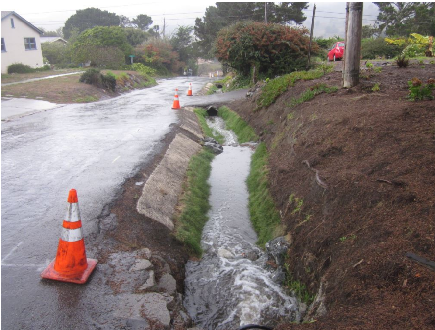
KAN001b-A_10312014: Farallone Ave @ 4 th St Post-construction
