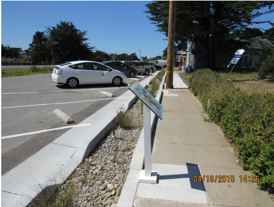
FITNEW1b-C_04162015: Carlos St Post-construction following installation of gravel, additional plants, wheel stops, and educational signs
