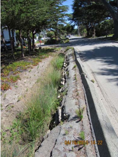
FITNEW1a-C_04162015: Wienke Way Post-construction additional planting
