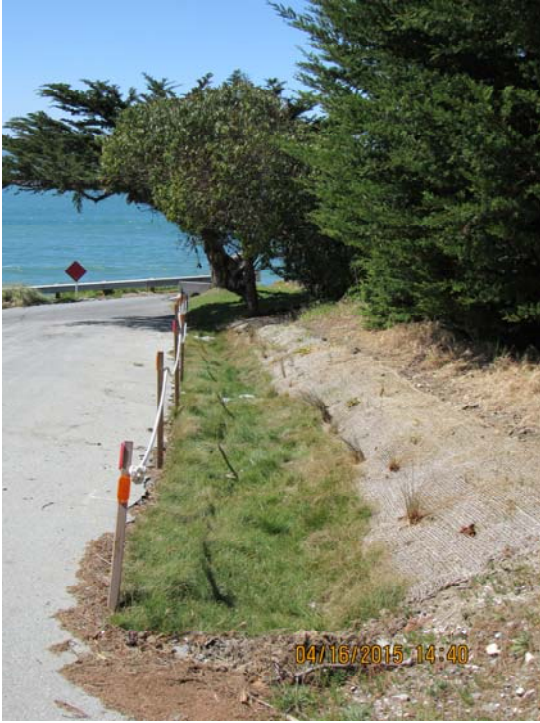
FIT002b-C_4162015: Seacliff Ct Post-construction additional planting
