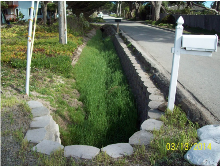
FITNEW1a-B_03132014: Wienke Way Post-construction
