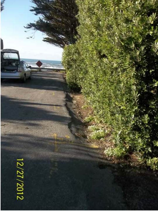
FIT024-A_12272012: Beach St Pre-construction
