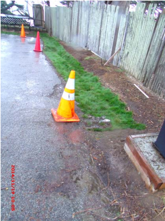
FIT006-B_11192014: 11 th St Post-construction
