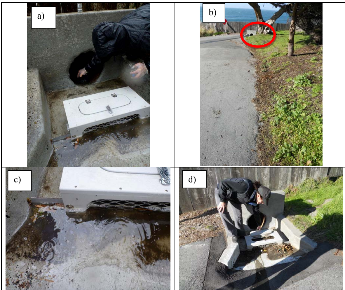
Figure 5. Flume filter at 6 th Street, Montara. Drainage area approximately 1 acre. A) Street runoff is channeled through flume filter before it enters the pipe discharging the water to the Reserve. B) Slope of street surface directs stormwater toward treatment spot (red circle). C) Oil and sediment are visible in stormwater before water flows through the BioMedia GREEN booms. D) After storms, sediment, leaves, and detritus need to be cleaned out of the filter box.
