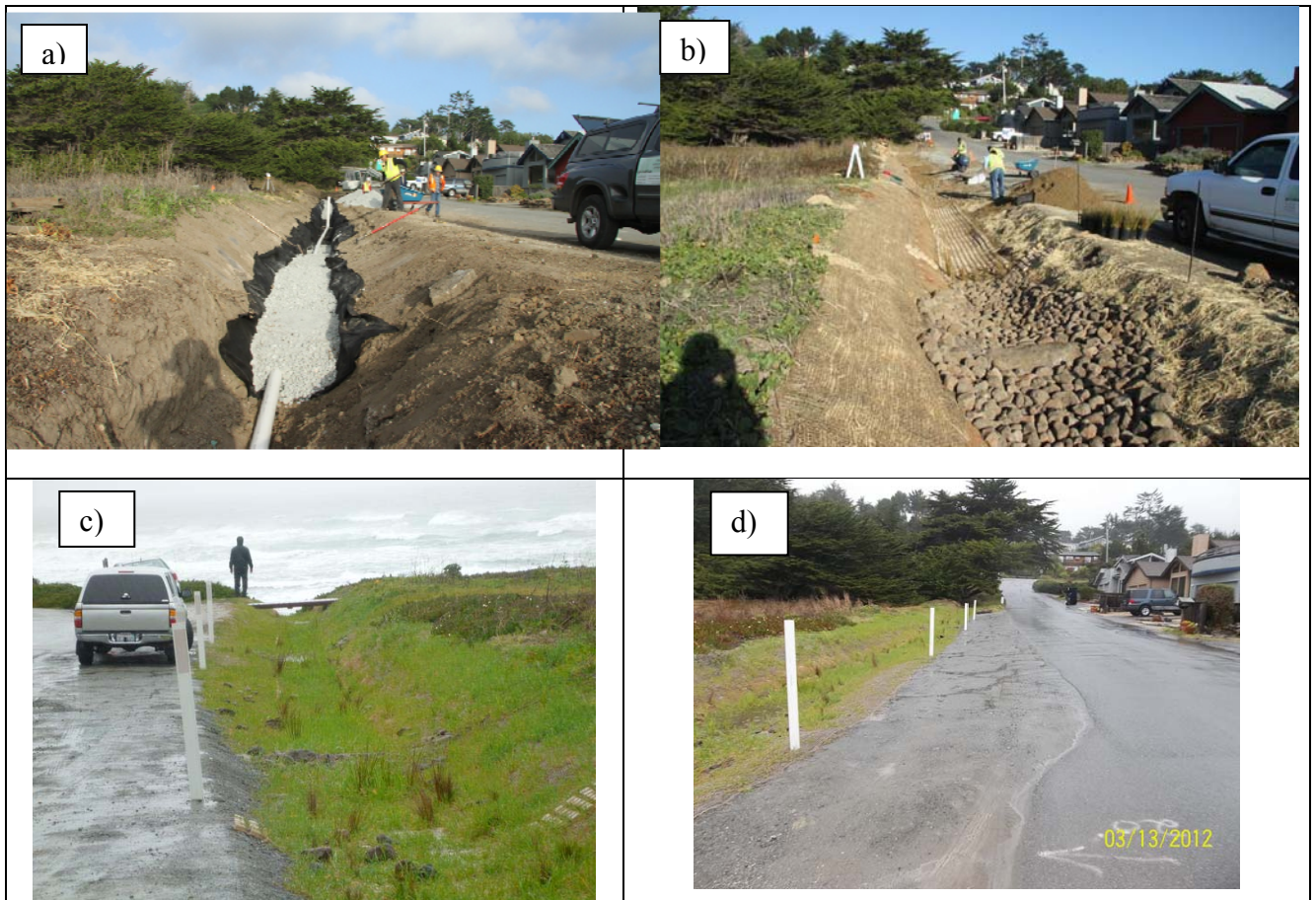
Figure 3. Vegetated swale at Juliana Ave., Moss Beach. Drainage area approximately 2.5 acres. A) Installation of filter fabric, drain rock and sub-drain. B) Installation of rock weirs and pavers. C) Finished swale looking west. D) Finished swale looking east. Stormwater enters swale at inlet on east end and from street surface between inlet and outlet.
