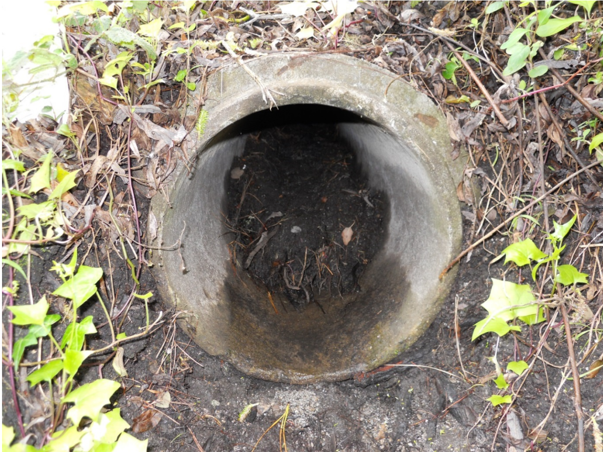
Figure 2. Outlet pipe discharging runoff after it has run through the cartridges. Sediment, seen here inside the pipe, from previous storms (before BMP installation) has likely accumulated contaminants.
