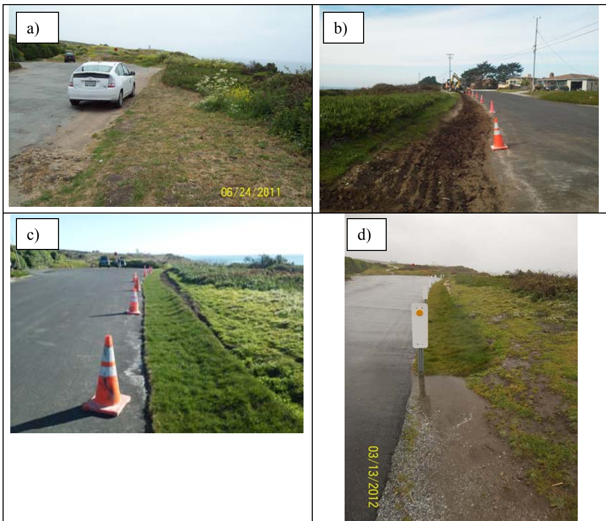
Figure 4. Grassy swale at Ocean Blvd., Moss Beach. Drainage area approximately 5 acres. A) Compacted area before beginning of construction. B) Installation of soil/compost mix after excavation. C) Installation of sod at the end of construction. D) Working swale during rainstorm.
