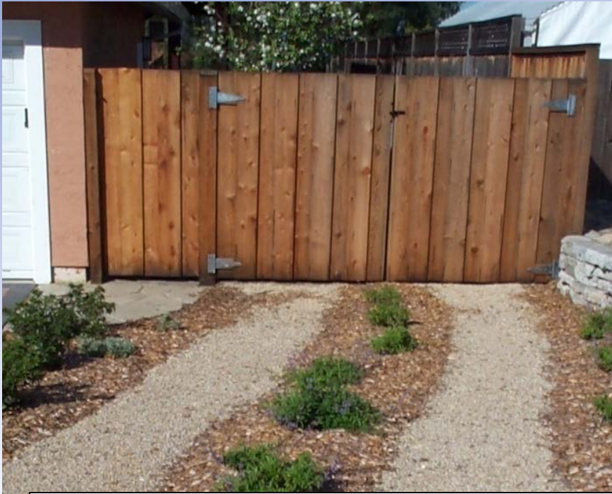
Plastic grid filled with gravel (two-track design)
