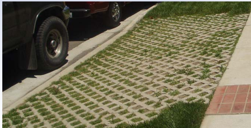
Example of Site Design Measure: Pervious paving.
