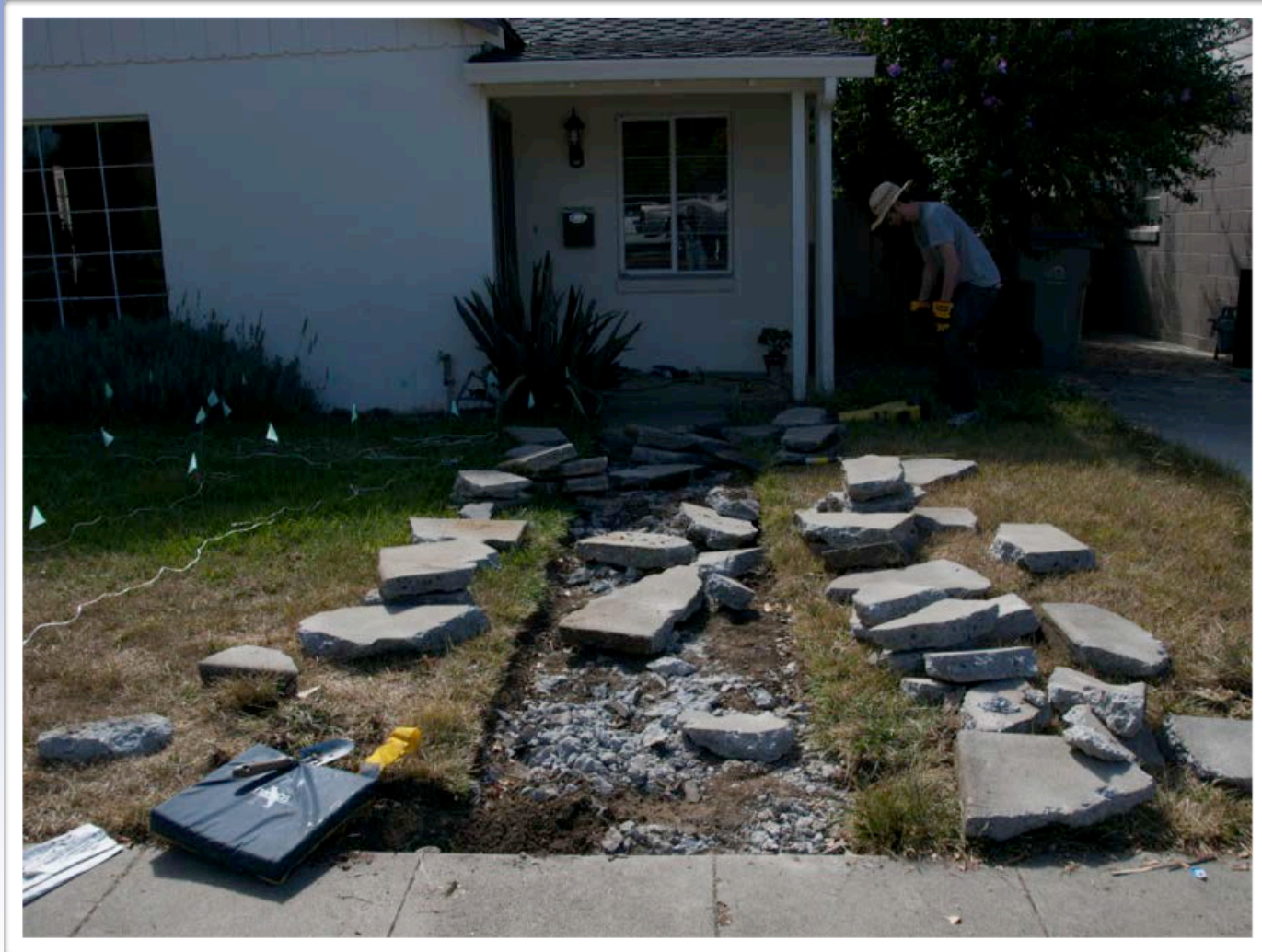
Jensen Residence, San Jose: Breaking up concrete
