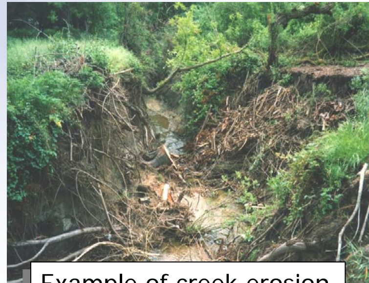
Example of creek erosion
