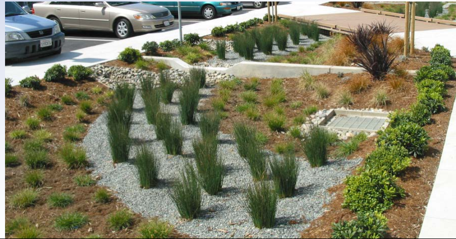
Example of Biotreatment: Bioretention area
